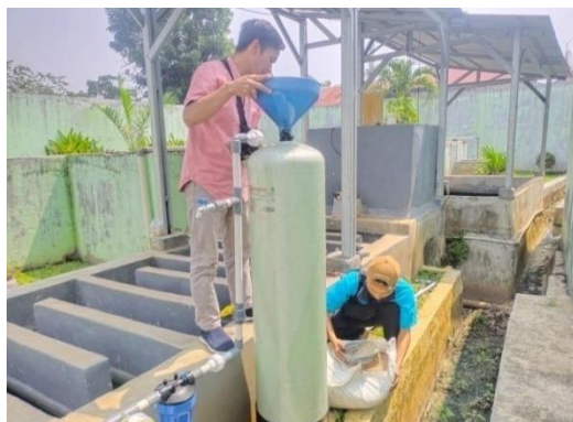
Figure 2. Filling silica sand in tubes
